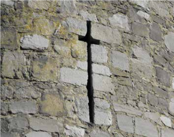
Crossform arrow loop in the south-west tower
